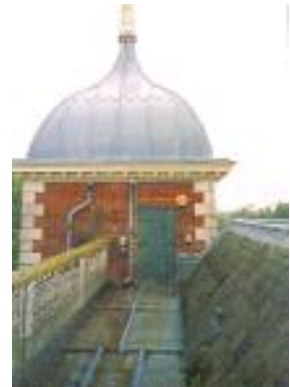
Part of the roof
